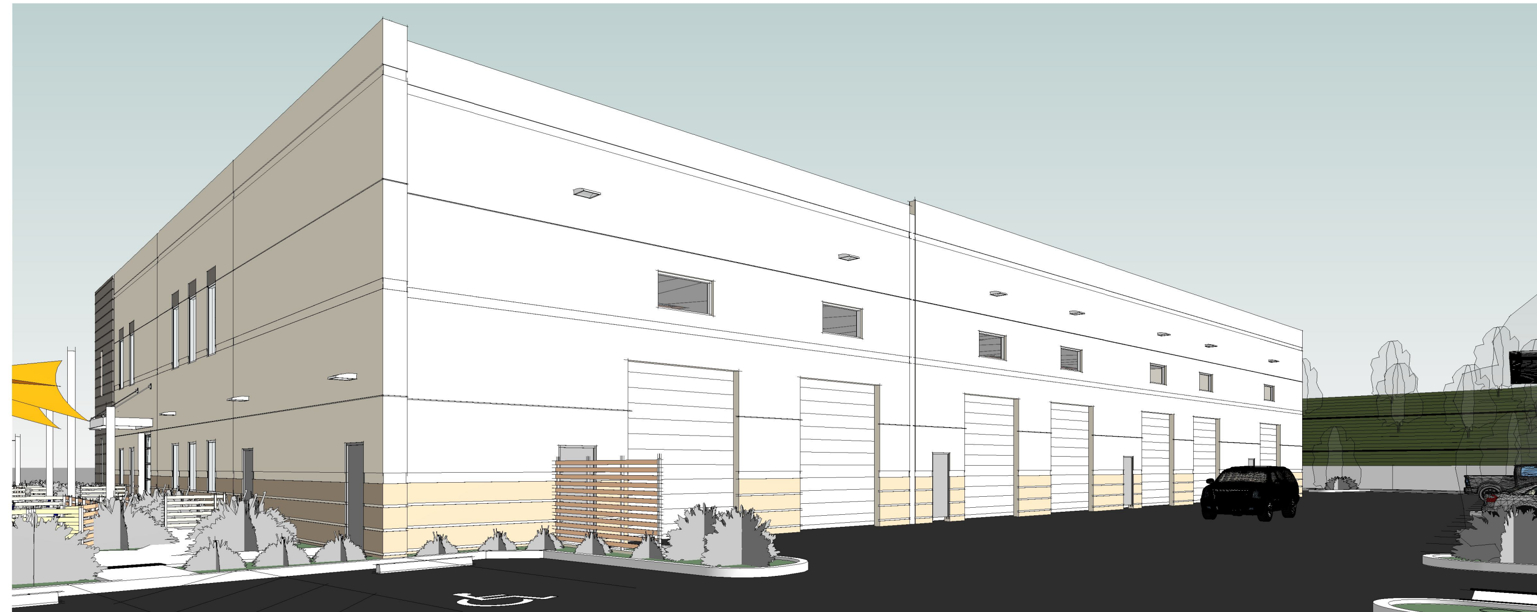
Building C SOUTHEAST CORNER
