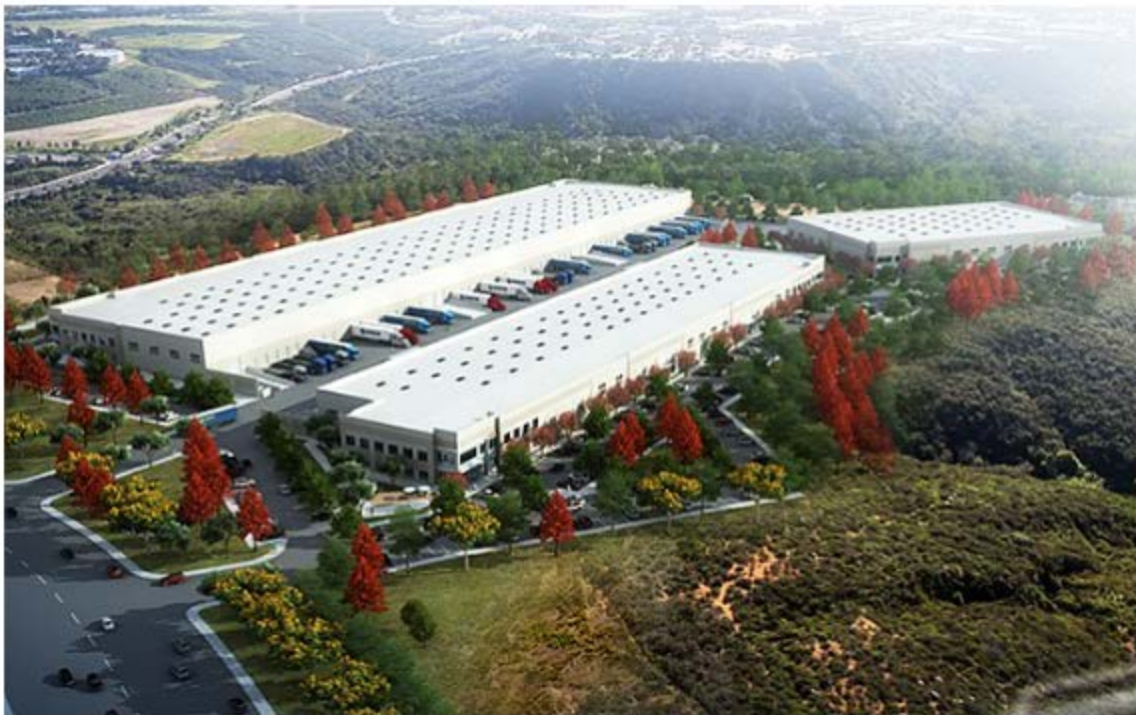
Rendering shows Ryan Cos. Pacific Vista Commerce Center in Carlsbad. Rendering courtesy of Ryan Cos.
