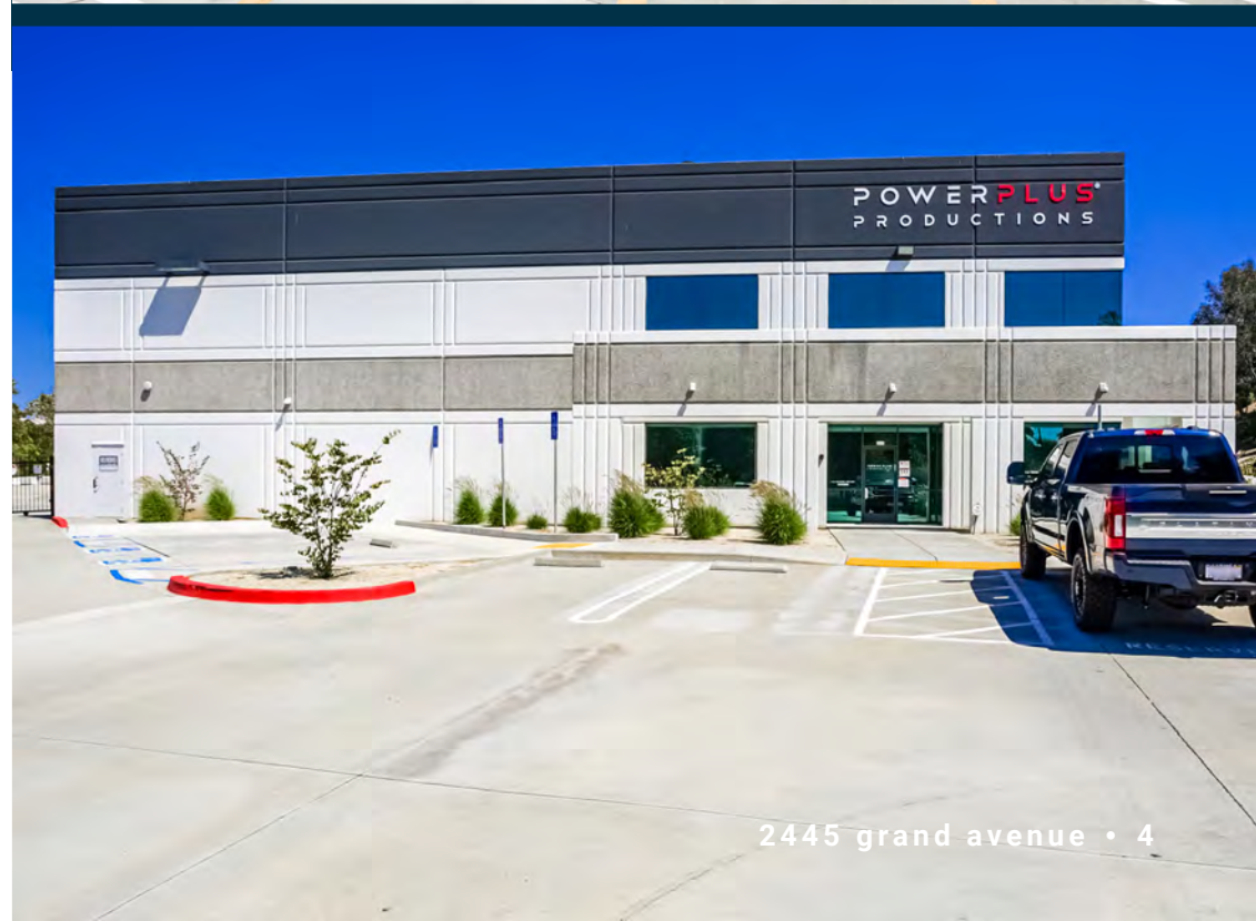
Dock & Grade Loading
