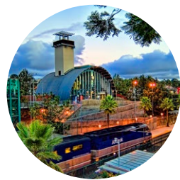
SOLANA BEACH TRAIN STATION
